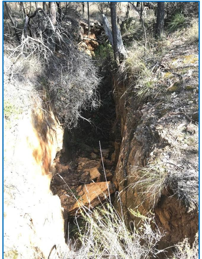
*Figure 3: Trench/costean type workings following the mineralised zone. The depth seems shallow, but the true extent cannot always be determined due to collapsed trench walls.*
