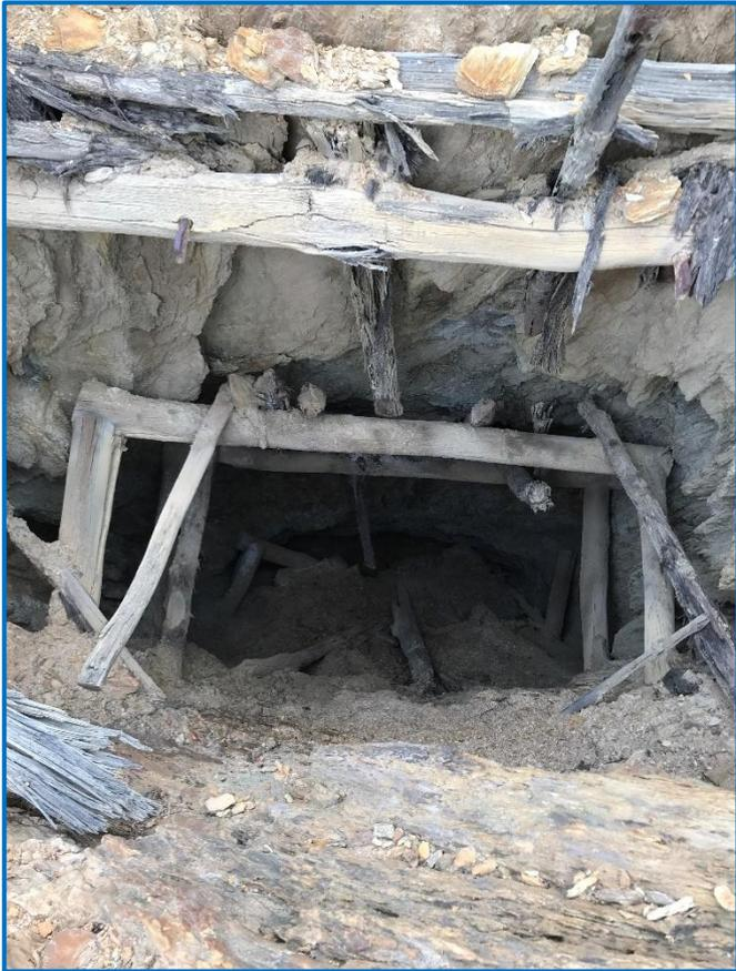
*Figure 2: Vertical shaft workings with timber supports toward the south western portion of the mapped area near the Tom's Lode workings.*
