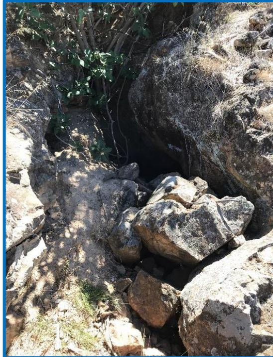
Figure 16: Collapsed adit entrance to the south of the shaft shown in Figure 15. Timber support can be seen deep inside the adit (not visible in the image).
