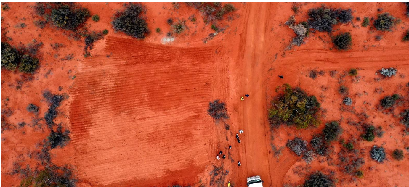
Figure 1: During the Quarter, the Ardea Team hosted the Consortium for meetings and also on-site visits to the KNP – Goongarrie Hub. Aerial image of work activities underway at the KNP – Goongarrie Hub, including water pump-testing “turkey nest” drill site rehabilitation on the left-hand side of the image.
