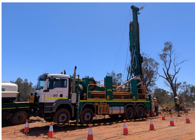
Figure 9: Diamond drilling is underway at the project
