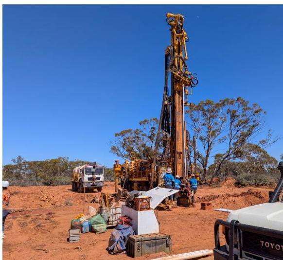
Figure 8: Hydrogeological well drilling is underway at the project
