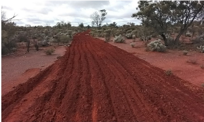
Figure 5: Example of early rehabilitation activities undertaken in 2026 at the Goongarrie Hub. All drill sample bags have been removed to a central “bag farm” and the drill rig access track scarified to promote expeditious understory regrowth.
